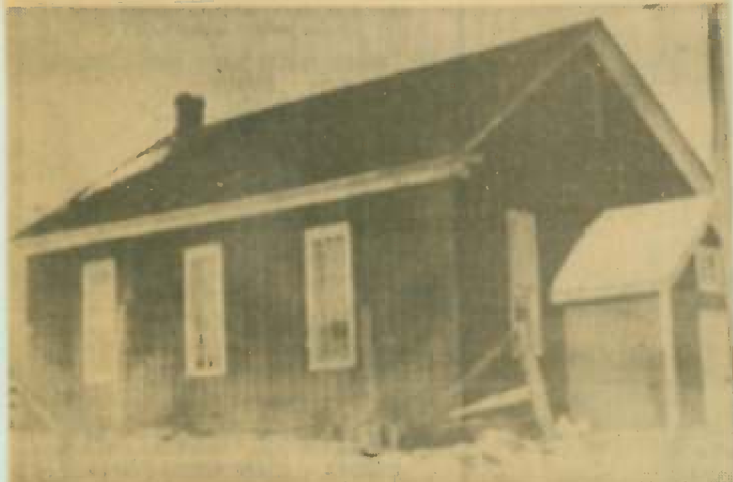
A cement step and a few wooden posts alone remain to mark the site where worshippers knelt in the old Daywood Church. It was demolished in 1937. It was a frame
